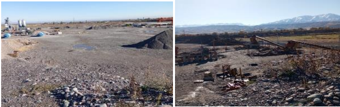
Figure 4. Dismantling equipment at production site.
